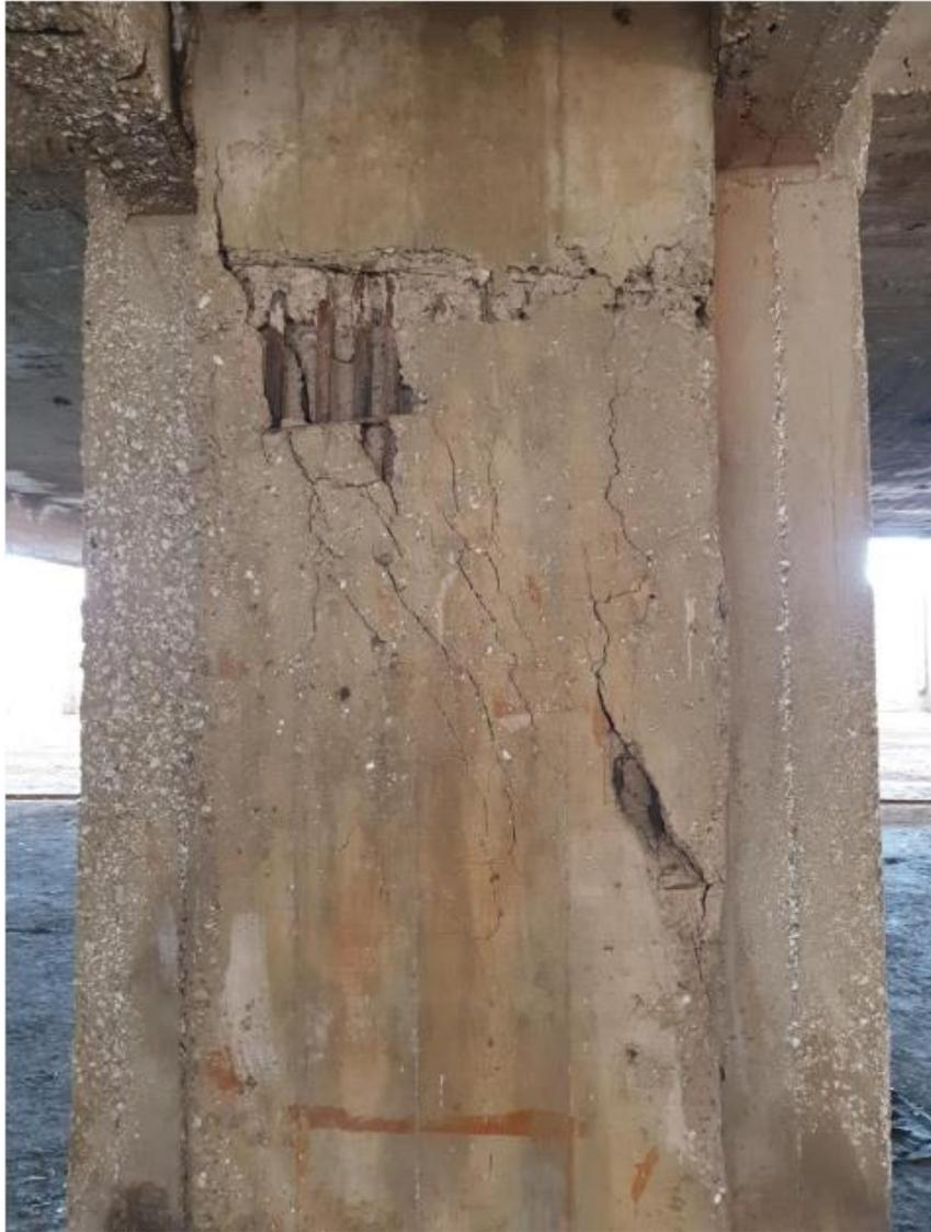
Figure 2.8. Column fire damage.
