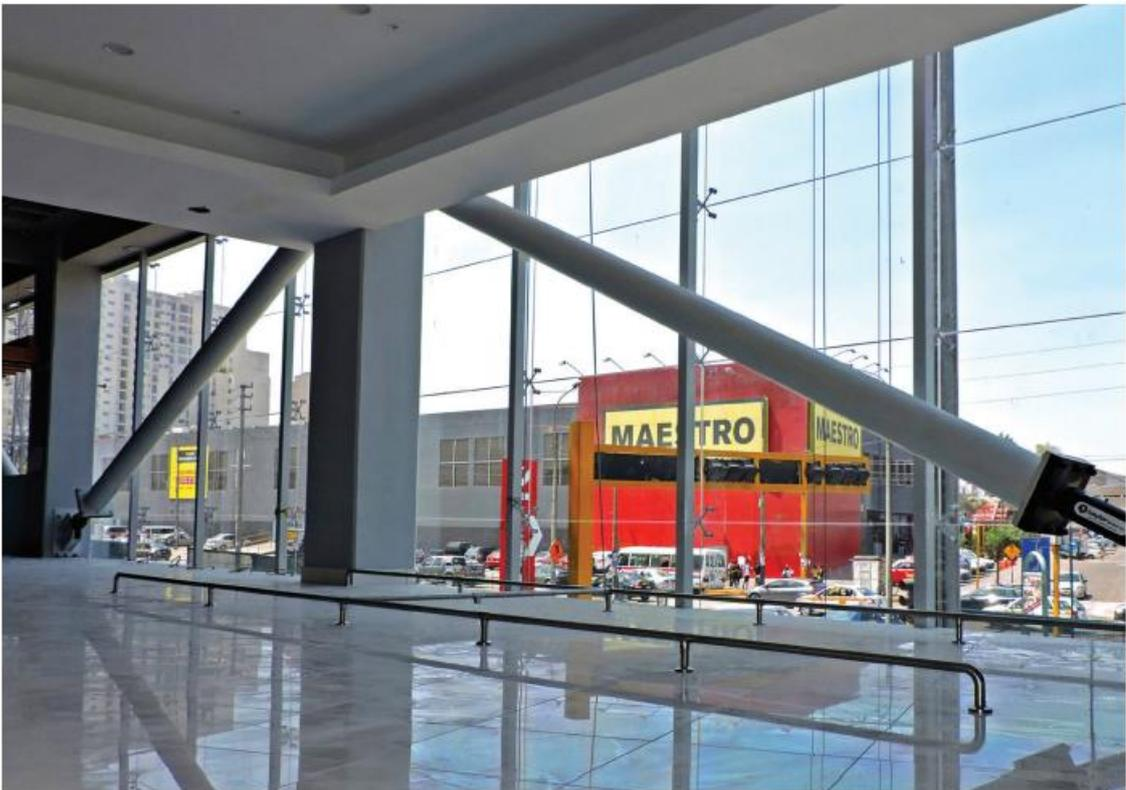
Figure 3.7. An example of diagonal bracing San Miguel Mall – Lima, Peru – New Build [33].
