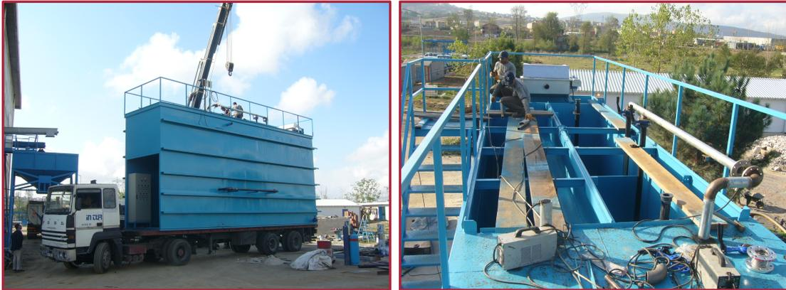
Figure 3.3. Atelier and on-site construction of the pilot unit.
