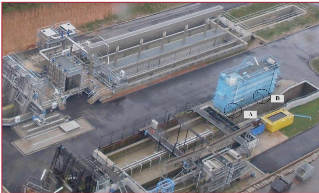
Figure 3.2. General overview of fine screens, grit chamber, Parshall flume and the pilot plant (A: Membrane permeate line B: Cloth filter permeate line).
