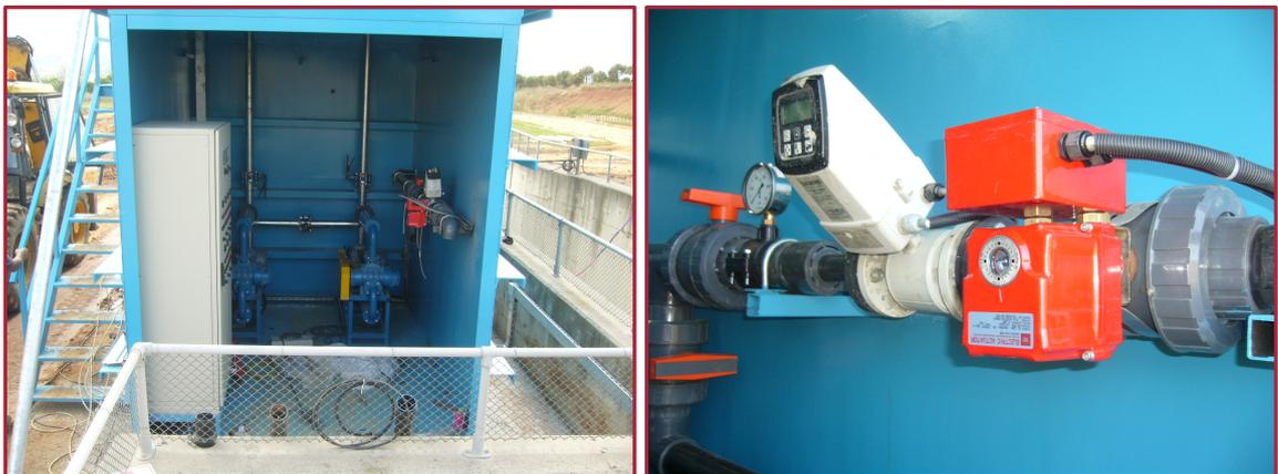
Figure 3.6. Control room: power panel, data logger, blowers and permeate instruments (left); permeate line in detail (right).
