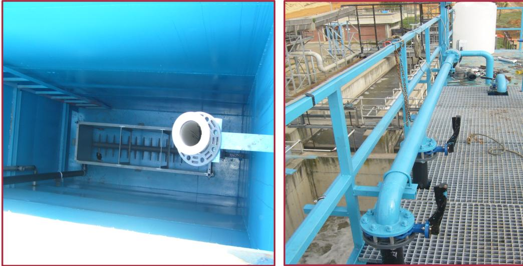
Figure 3.5. Coarse bubble diffusers (left) and diffuser piping (right).
