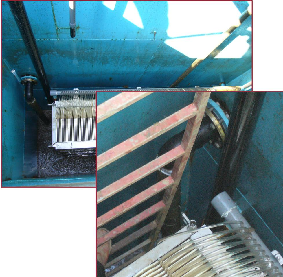
Figure 4.1. Stabilised cake layer on the cloth filter.
