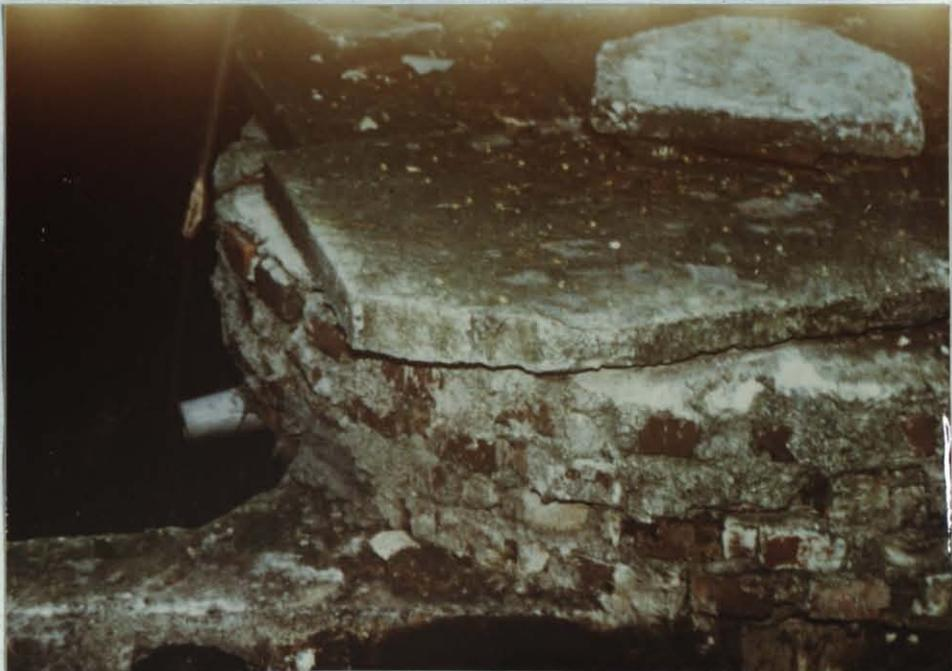
Figure 7 : Photograph of the Inlet Tank "L" Type Covering Plate and Overflow pipe
