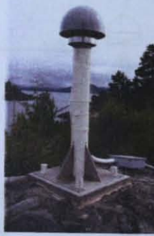
Figure 3.15. Sample of Steel Pillar for fully rocky surfaces
