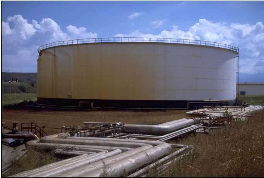
Figure 2.2. Diamond shape buckling at the upper part of the tank shell (Kocaeli Earthquake of 1999)
