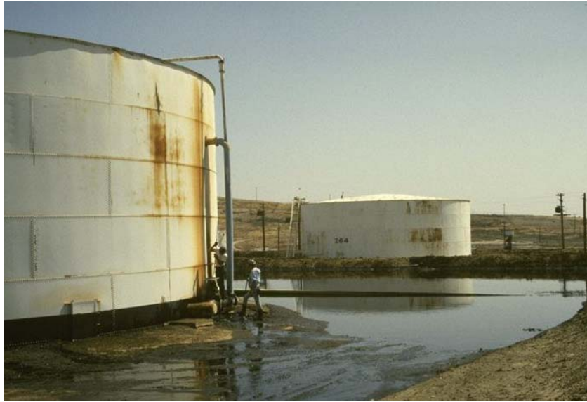
Figure 2.8. Broken pipe connections (Coalinga Earthquake of 1983)
