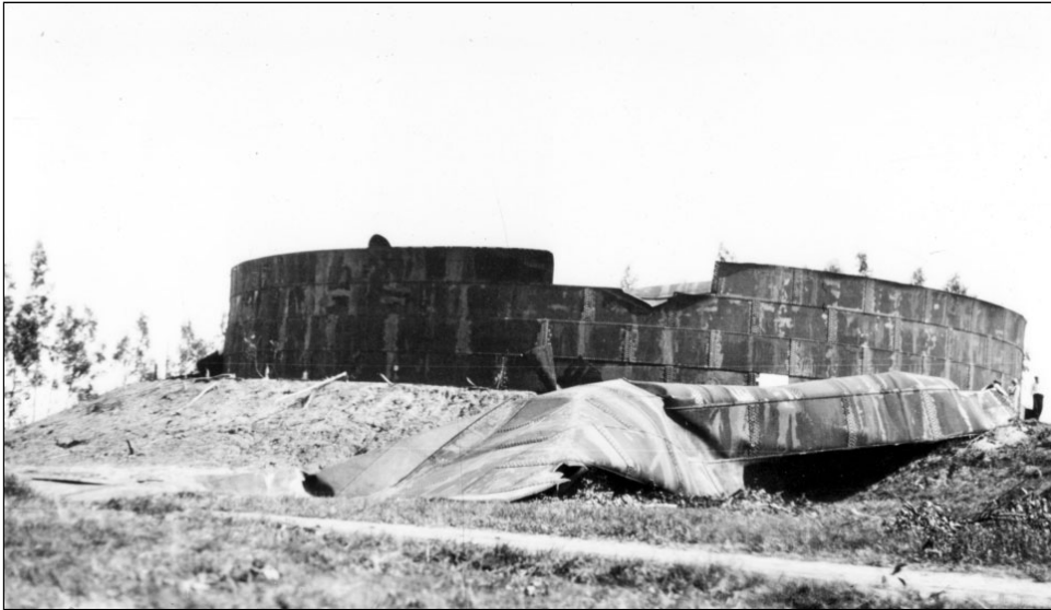
Figure 2.6. Sloshing damage to a water storage tank (Long Beach, California Earthquake, 1933. Courtesy of Harold M. Engle)
