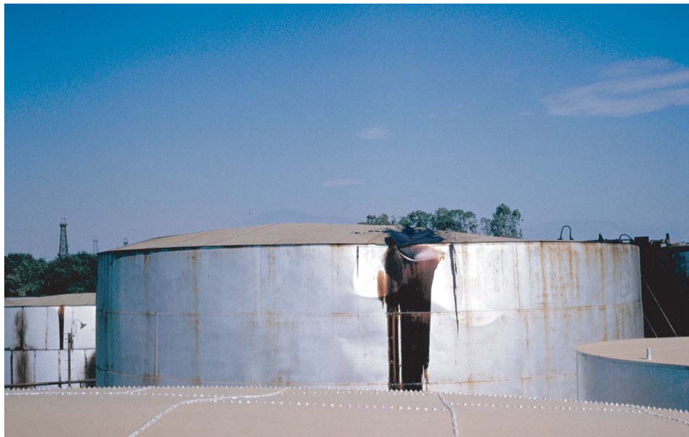
Figure 2.5. Sloshing damage to an oil tank (Kern County, California Earthquake, 1952) (courtesy of K. V. Steinbrugge)
