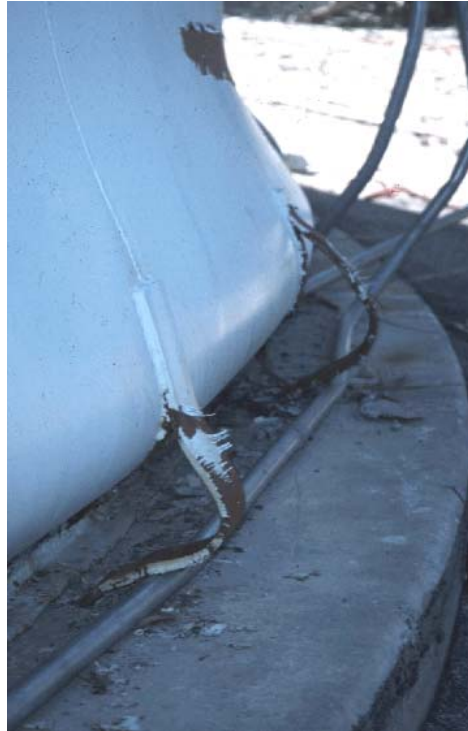
Figure 2.4. Elephant foot buckling damage of Santa Clarita Valley tank (Northridge Earthquake, 1994)
