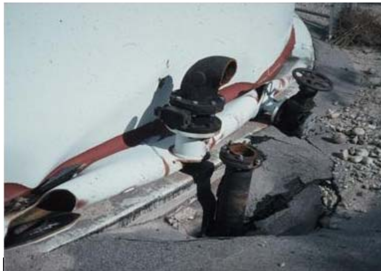
Figure 2.7. Piping break and shell buckling
