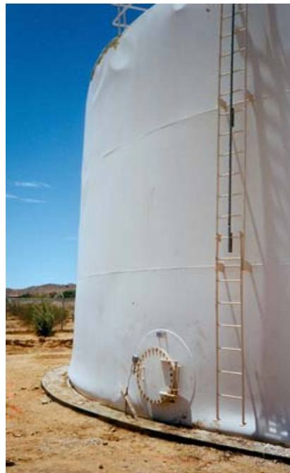
Figure 2.3. Elephant foot buckling damage of a water tank (Landers Earthquake)
