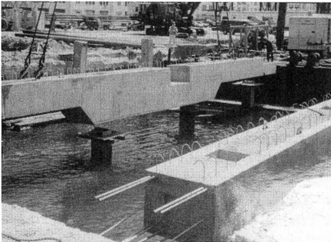
Figure 4.13. Precast concrete pile-cap (Port Engineering, 2004)
