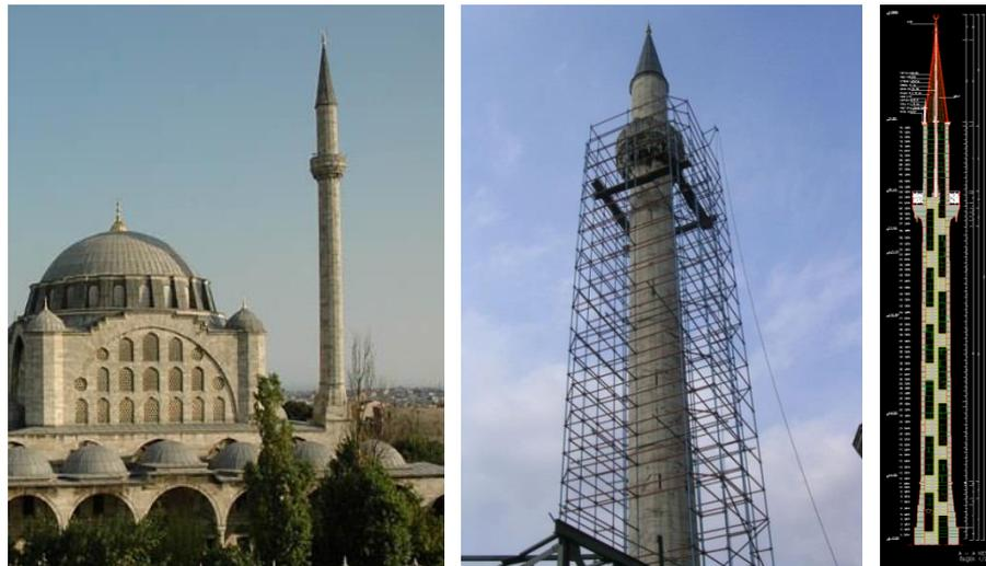
Figure 4.2. Images of the Mihrimah Sultan Mosque (left), its minaret before its disassemblage (center), cross-section of the minaret (right).
