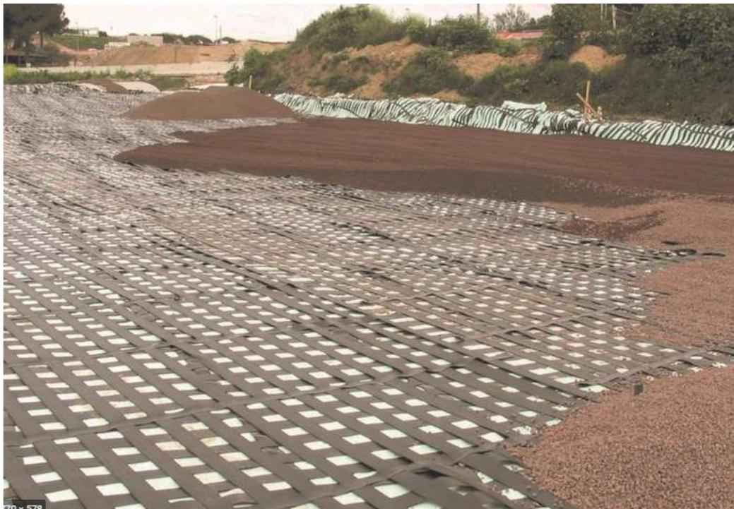
Figure 2.2. Soil Reinforcement with Geosynthetic (Geosyntheticsmagazine, 2019).
