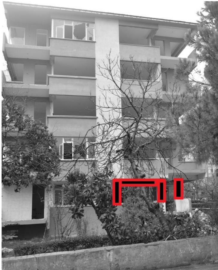
Figure 6.1. The reinforced concrete building investigated and the structural elements removed to induce damage.
