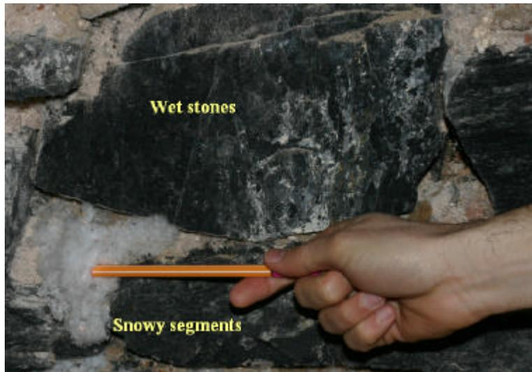
Figure 3.2. High humidity over stones and its effects
