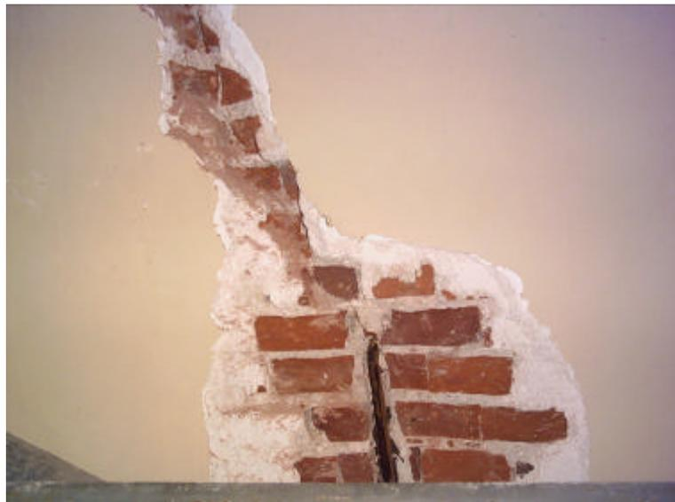
Figure 3.9. Masonry configuration in the stair case of harem
