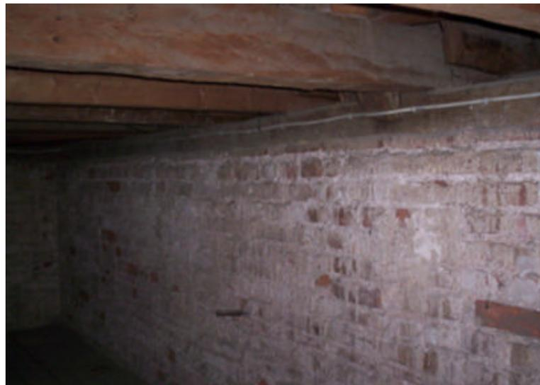
Figure 2.15. Structural wall and timber slab in the roof of the structure
