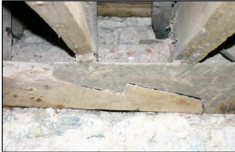
Figure 2.14. Splice of timber beam between the structural wall and slab girders
