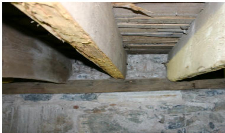
Figure 3.3. Chipped timber beams due to decay on the foundation floor
