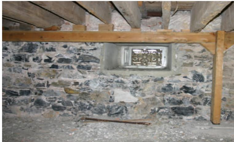
Figure 3.1. Ventilation opening in the foundation floor
