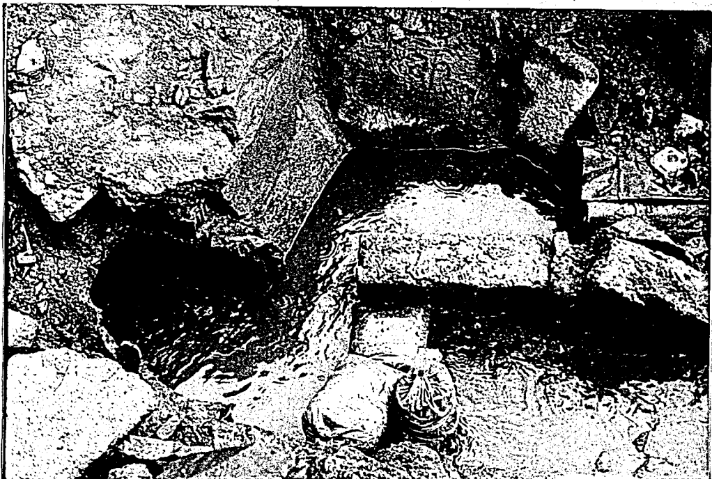
8- Diverted sewer into the galvanized pipe.
