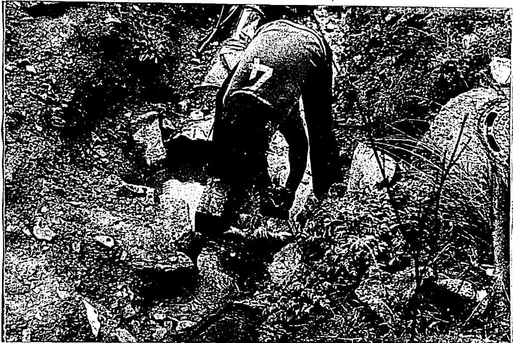
7- Blocking the sewer outfall by sand-bags and diverting the sewer into the galvanized pipe.
