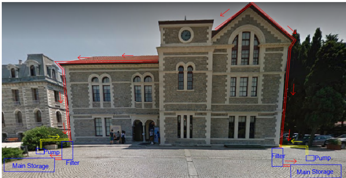
Figure 4.16. Rainwater harvesting systems in Albert Long Hall.
