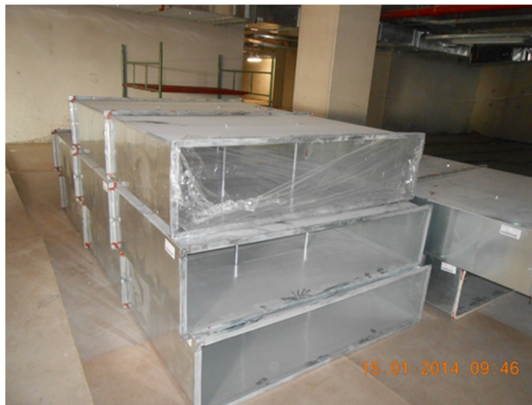
Figure 4.14. Sealing ductwork.
