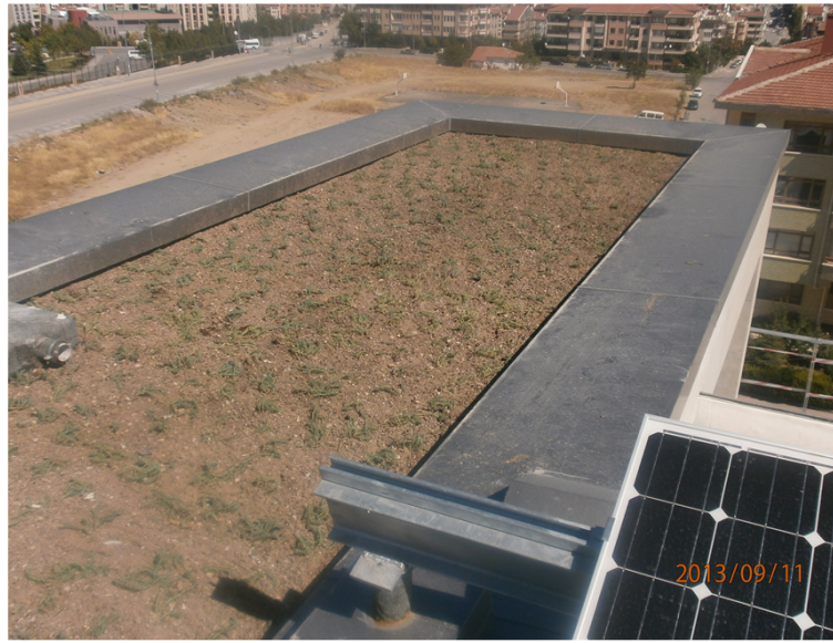
Figure 4.31. Green roof implementation of Case 2.
