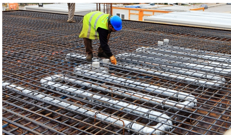
Figure 4.35. Duckwork inside the slab.
