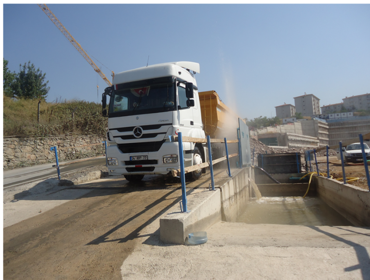
Figure 4.7. Truck washing area of Case 1.
