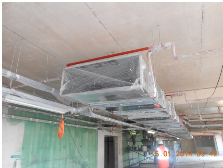
Figure 4.15. Sealing ductwork.
