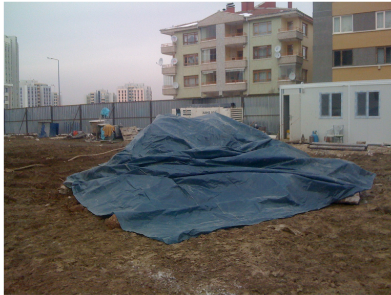
Figure 4.25. Protection of Sand Stockpile in Case 2.
