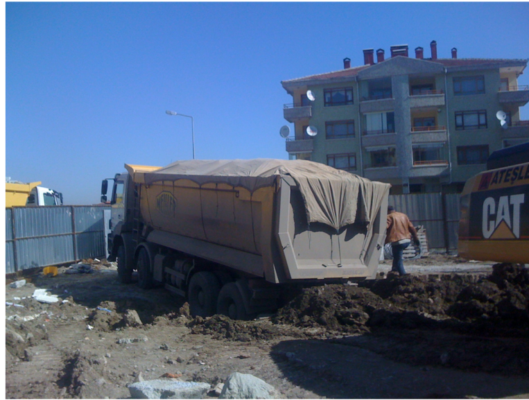
Figure 4.27. Truck covering of Case 2.
