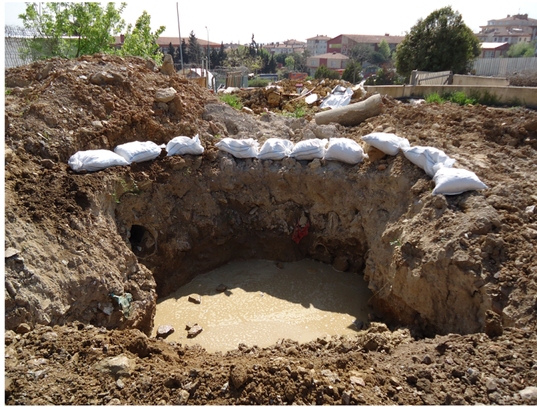
Figure 4.6. Sediment trap of Case 1.
