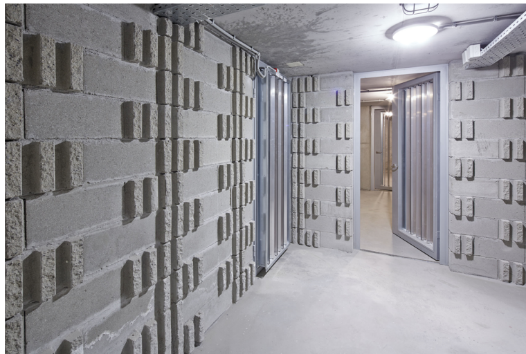
Figure 4.33. Photograph of air labyrinth.
