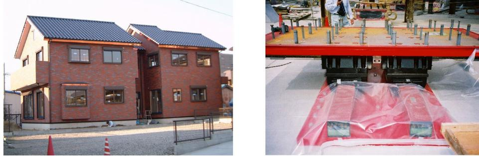
Figure 2.7. Seismically Isolated Japanese Private House and Recentering Devices (Martelli & Forni, 2010).
